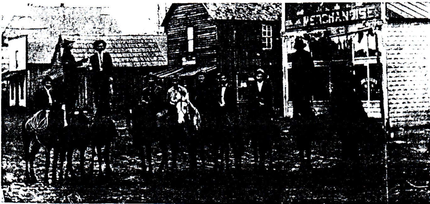
North side of Main Street in Kansas, Oklahoma—1913 Reading left to right: Bank, Neal Cayce's Barber Shop [white front], McGowan's Cafe, Post Office [sign above porch roof], Pitts Store [later Jim Pifer and now Community Church.
